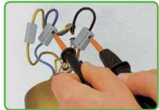
Testing through separate test slot.
